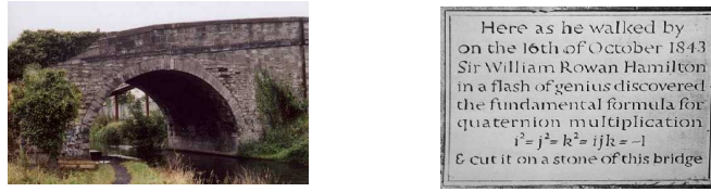
FIGURE 888. Brougham Bridge in Dublin
